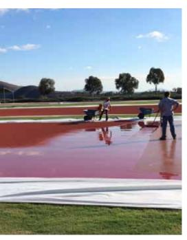
The 400-meter, eight-lane, polyurethane running track with a 12-lane, 100-meter straightaway and an infield area for jumping events, is
